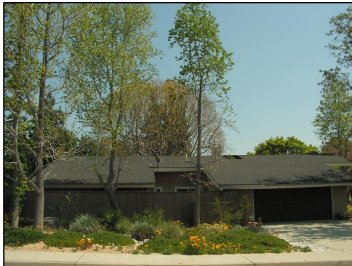
Figure 2: Eliminate the vertical and horizontal continuity. This is a good example of adequate separation.
